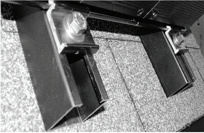
Figure 8a: Mounting Clips for Flush Mount
